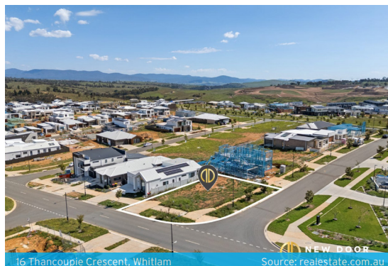
16 Thancoupie Crescent, Whitlam
