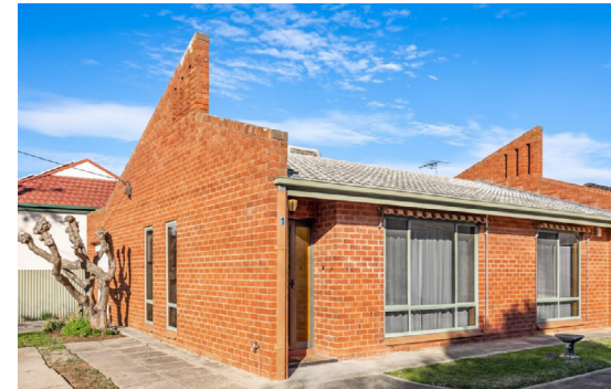
1/29 Ormond Avenue, Daw Park Source: realestate.com.au
