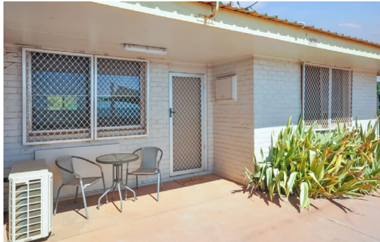
Sutherland Street, Port Hedland
