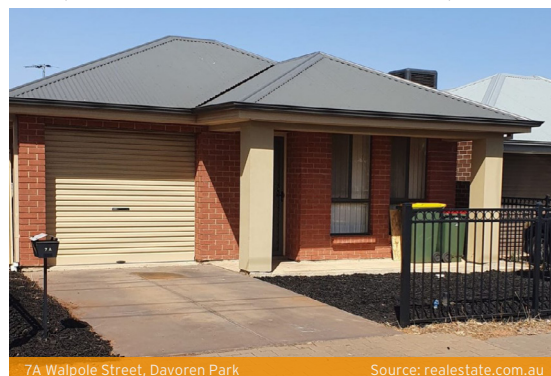
7A Walpole Street, Davoren Park Source: realestate.com.au
