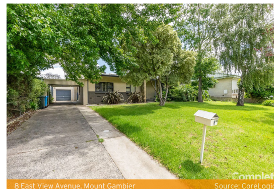
8 East View Avenue, Mount Gambier Source: CoreLogic
