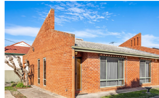
1/29 Ormond Avenue, Daw Park Source: realestate.com.au
