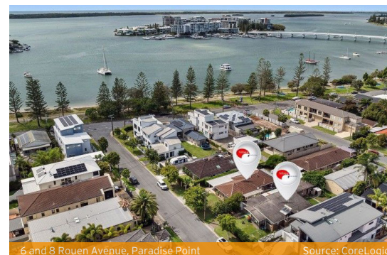
6 and 8 Rouen Avenue, Paradise Point
