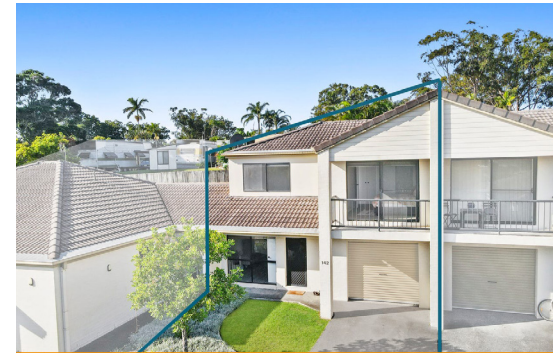
142/590 Pine Ridge Road, Coombabah
