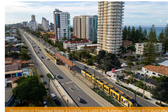
Illustration of Proposed Stage 3 Gold Coast Light Rail Extension Source: RCP Australia
