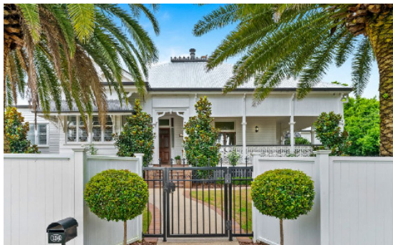
136 Mackenzie Street, East Toowoomba
