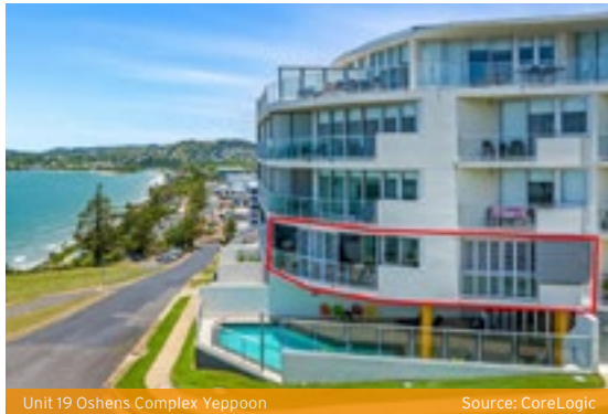
Unit 19 Oshens Complex Yeppoon
