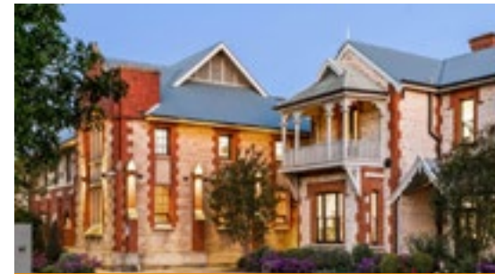
64 North Terrace, Kent Town Source: realestate.com.au
