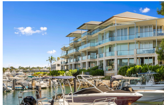
44/1 Corkhill Street, North Fremantle
