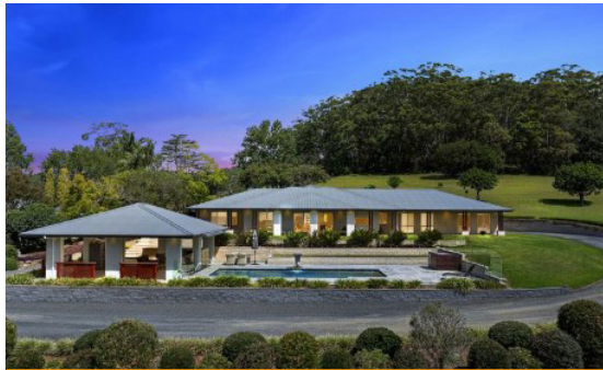
336 Yarramalong Road, Wyong Creek
