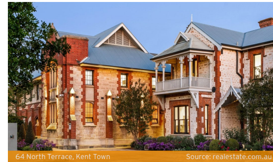
64 North Terrace, Kent Town Source: realestate.com.au
