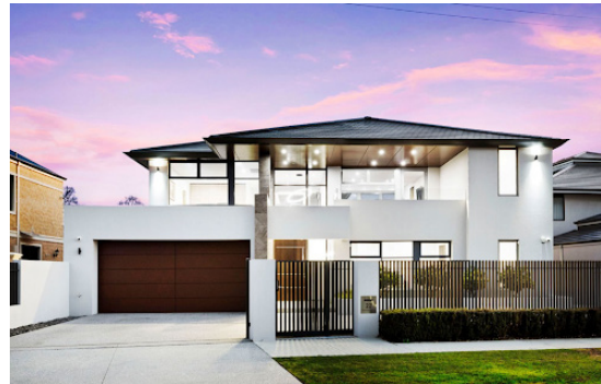
22 Swanview Terrace, South Perth
