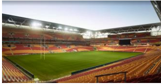
Brisbane Stadium 'Suncorp Stadium'
