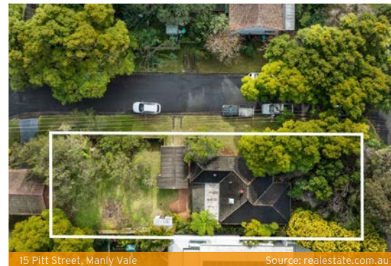
15 Pitt Street, Manly Vale Source: realestate.com.au
