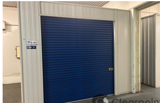
312/23-27 Mars Road, Lane Cove West Source: realcommercial.com.au
