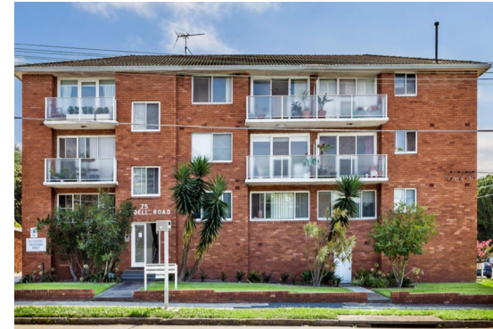
8/73-75 Wardell Road, Dulwich Hill Source: realestate.com.au
