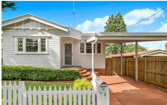
14 George Street, East Toowoomba
