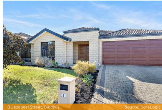
8 Jezabeel Street, Baldivis
