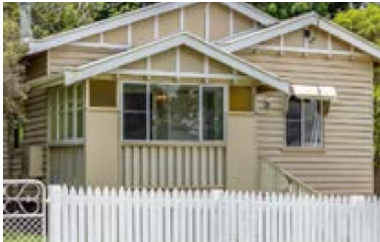
4 Atkinson Street, South Toowoomba
