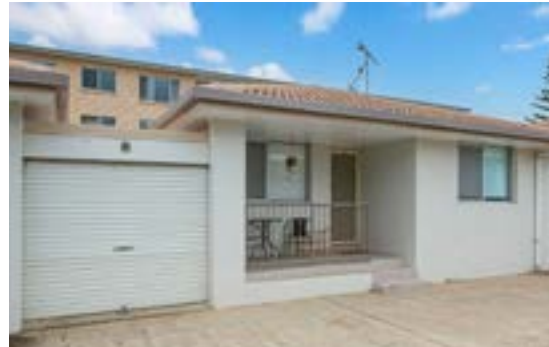
3/30 Seaview Street, Kingscliff Source: CoreLogic
