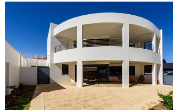
96 Kempton Street, Bluff Point
