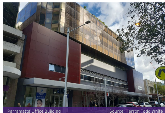
Parramatta Office Building
