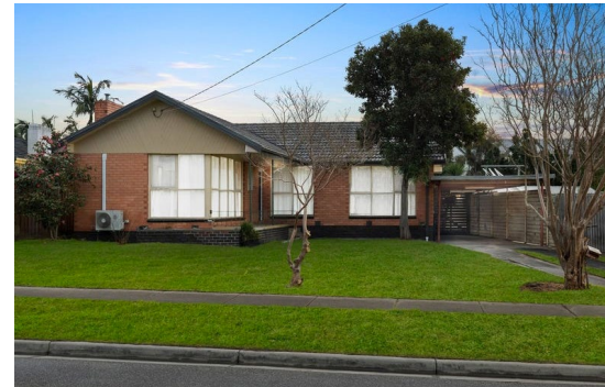
1 Parkland Avenue, Hampton Park Source: realestate.com.au
