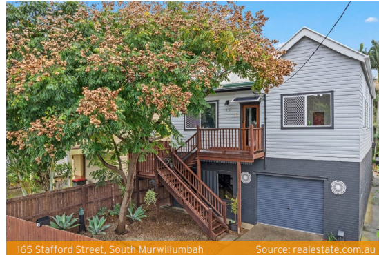
165 Stafford Street, South Murwillumbah Source: realestate.com.au
