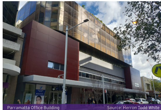
Parramatta Office Building
