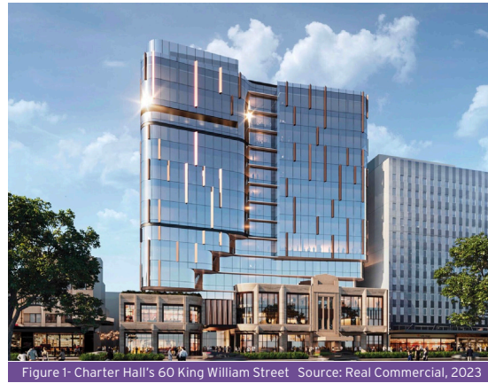
Figure 1- Charter Hall's 60 King William Street Source: Real Commercial, 2023
