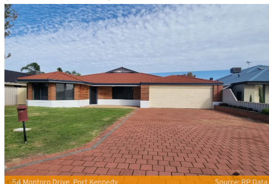
54 Montoro Drive, Port Kennedy
