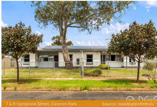
7 & 9 Yarnbrook Street, Davoren Park Source: realestate.com.au
