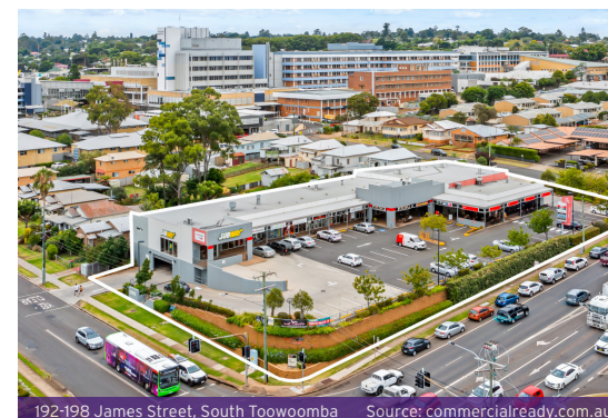
192-198 James Street, South Toowoomba Source: commercialready.com.au
