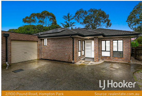
2/100 Pound Road, Hampton Park Source: realestate.com.au
