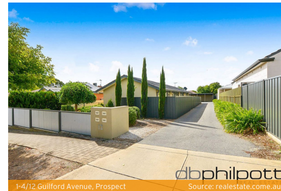
1-4/12 Guilford Avenue, Prospect Source: realestate.com.au
