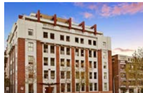
513/105 Campbell Street, Surry Hills
