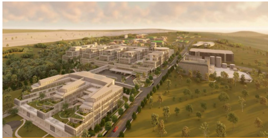
Toowoomba hospital site
