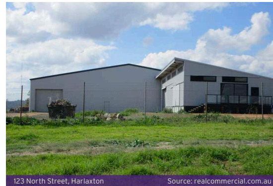
123 North Street, Harlaxton Source: realcommercial.com.au
