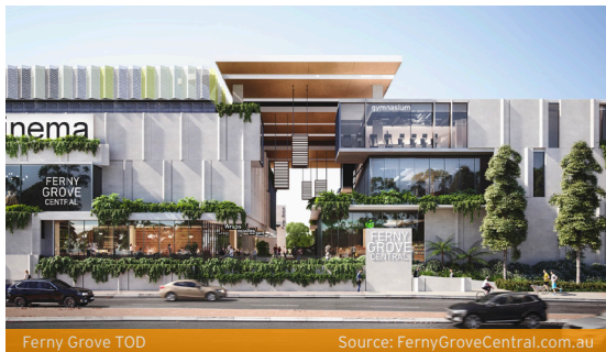
Ferny Grove TOD Source: FernyGroveCentral.com.au
